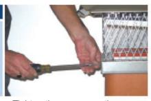
Tighten the screws on the capdamper just like on a chimney cap.
