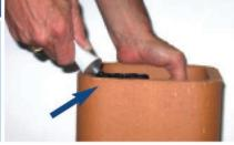
To achieve a total seal, first run a thick bead of silicone around the flue liner top.
