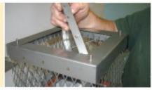
Angle damper and pull through frame, the flue is now ready for brushing.
