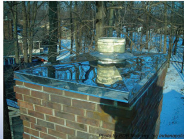
New Stainless Steel chase is rust resistant and functions properly for years of safe operation.
